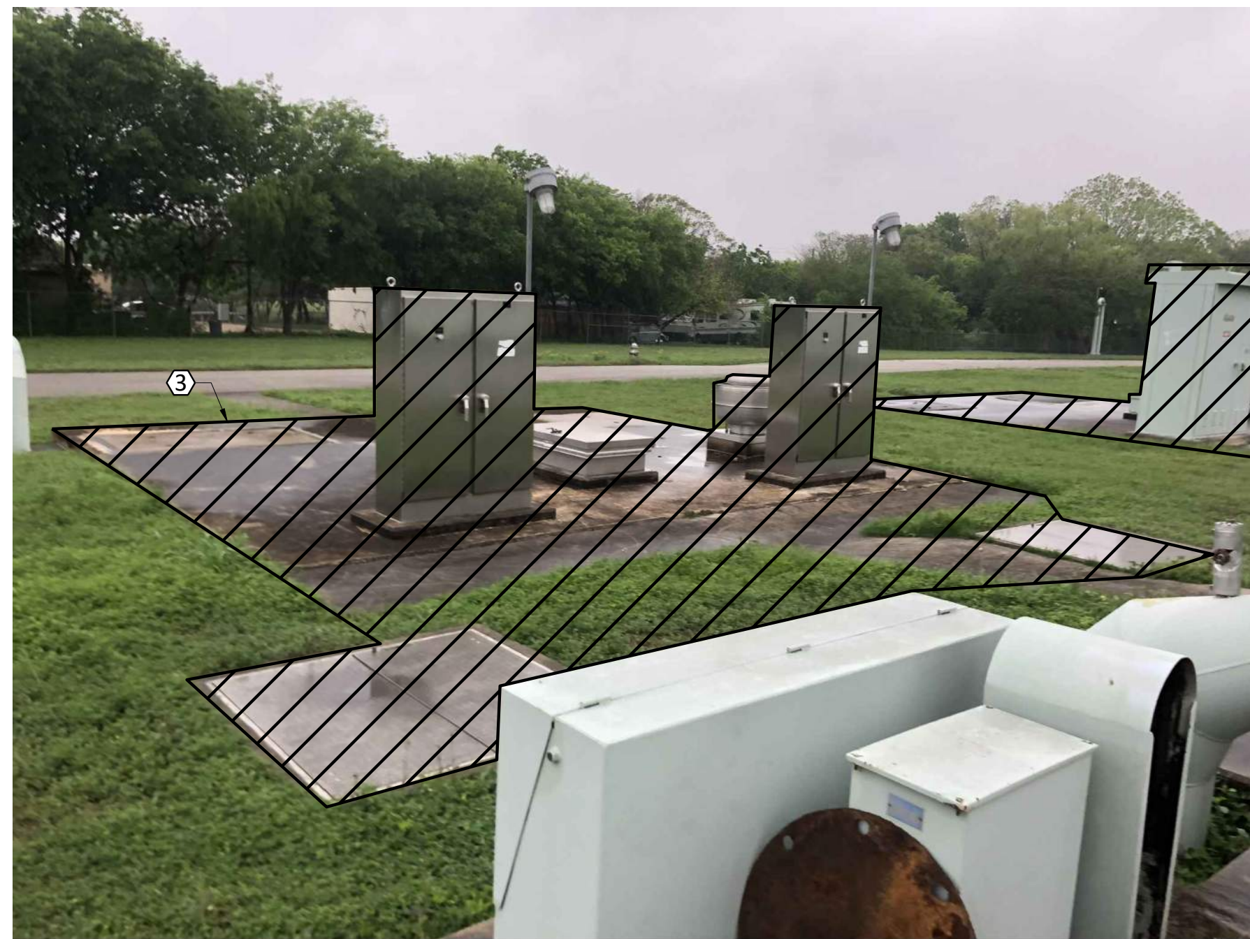
3 - EXISTING HSP 1-4 AND HSP 2-4 DISCHARGE VALVE VAULTS DEMOLITION
