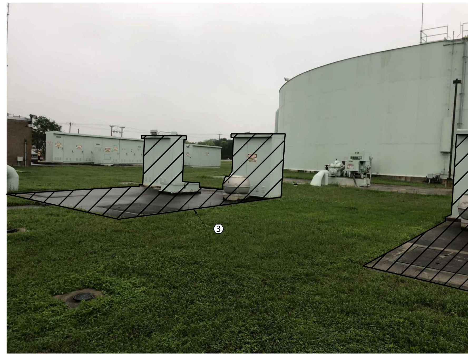
2 - EXISTING HSP 1-6 AND HSP 2-6 DISCHARGE VALVE VAULTS DEMOLITION
