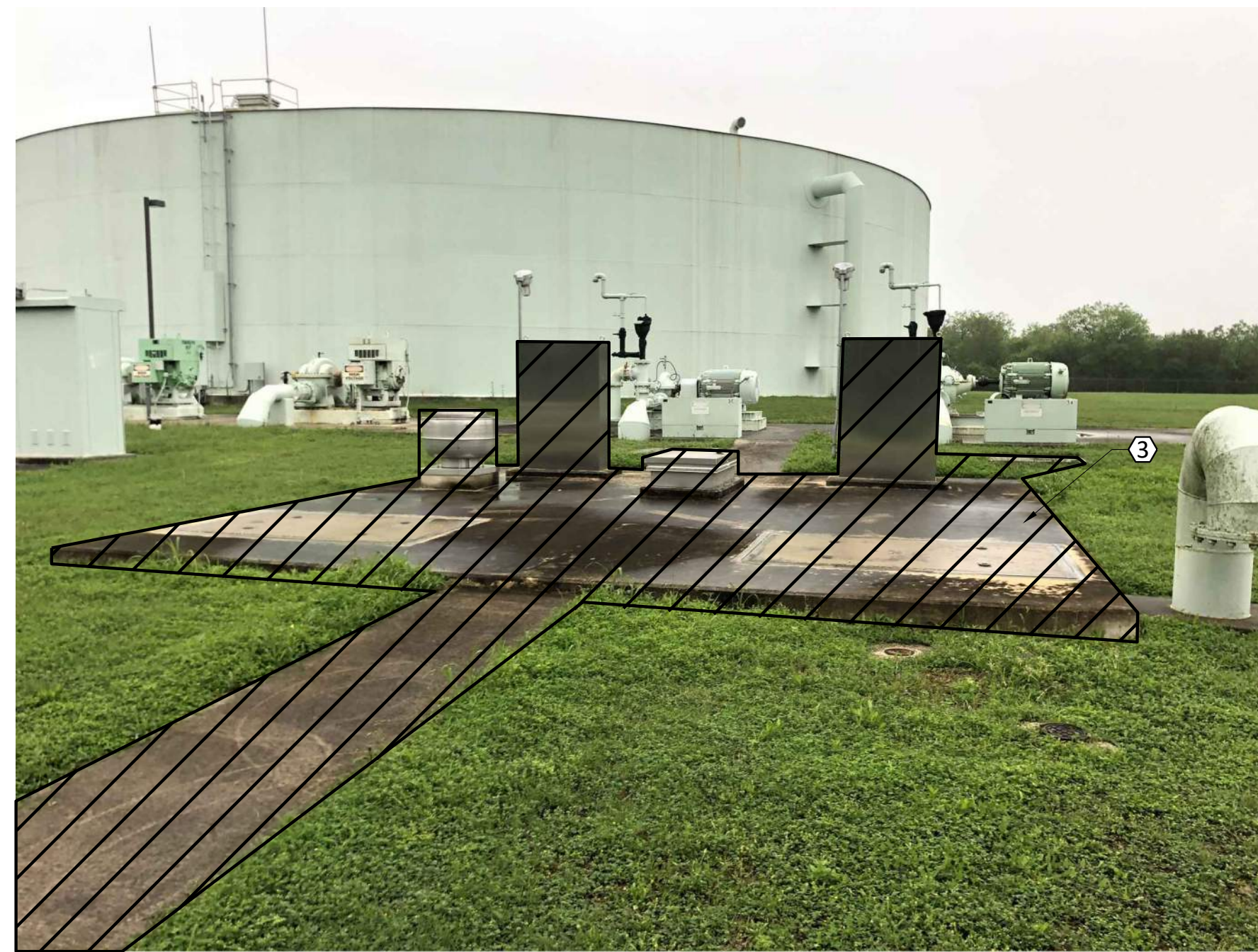
2 - EXISTING HSP 3-6 AND HSP 3-4 DISCHARGE VALVE VAULTS DEMOLITION
