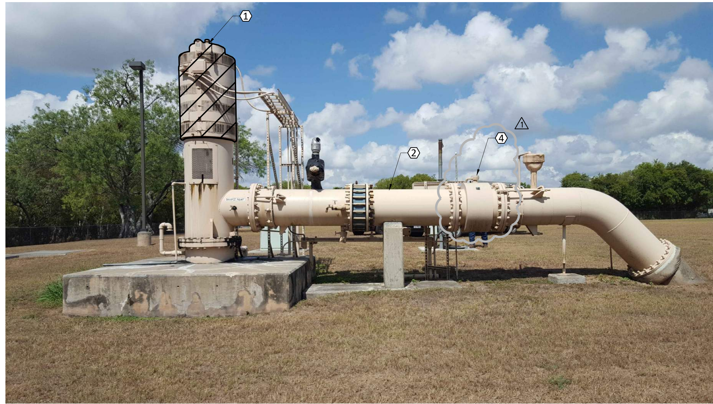
1 - EXISTING WELL NO.3 DEMOLITION
